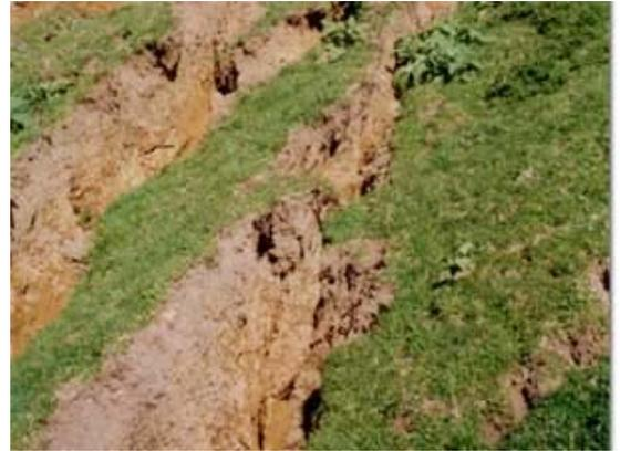
**Slope failure showing ruptured ground and tension cracks.**
